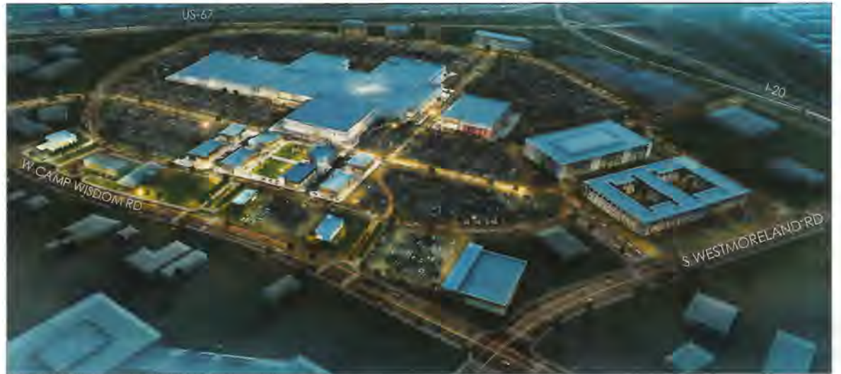
Palladium RedBird is 50 percent constructed right now but 60 percent preleased. The project, a redevelopment of the former Red Bird Mall on the south side, is a public-private partnership between Dallas Housing Finance Corp. and Dallas-based Palladium USA.
