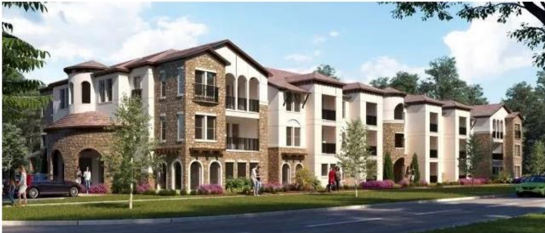
The Palladium East Berry Street apartments are being built near Fort Worth's medical district. (Cross Architects )
