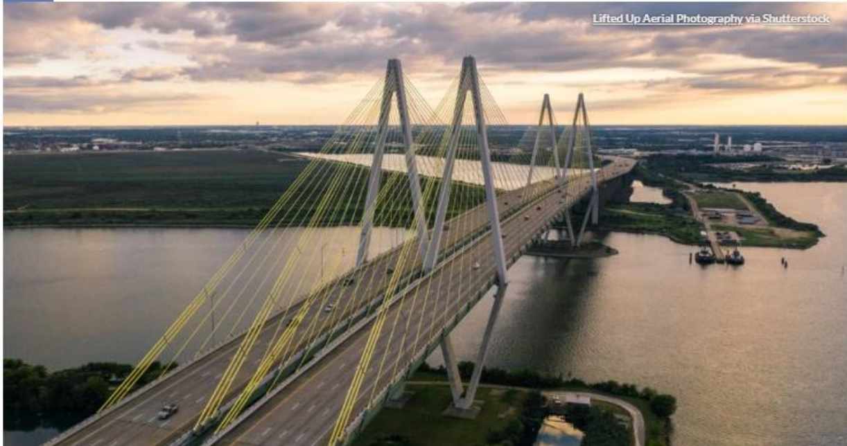
Aerial view of Fred Hartman Suspension Bridge in Baytown, Texas
